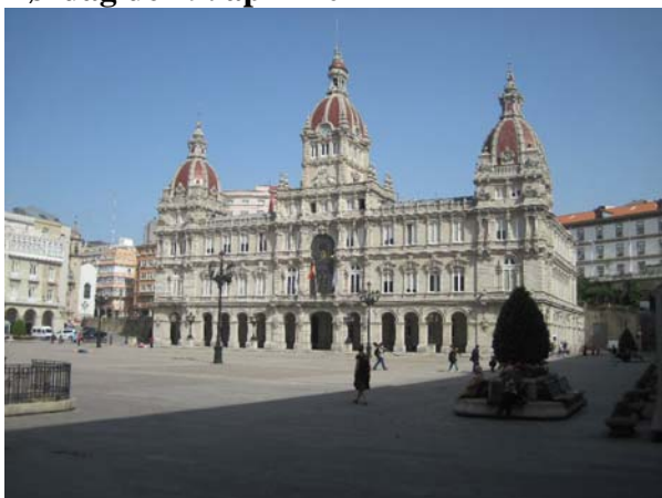
Plaza Mayor i La Coruña
